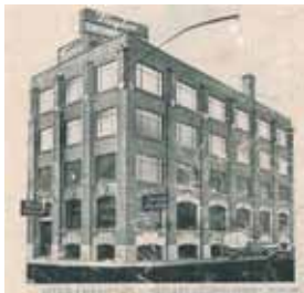
Office and manufacturing plant, Church St, Toronto 1934
